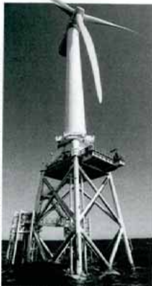
The underground power cable will transport electricity from wind turbines in the outer Moray Firth to Inverboyndie and on to two new sub-stations near New Deer.
