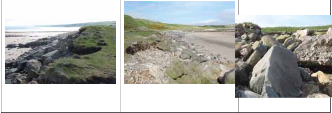
Plate 4.3 Boulder rock armour on the western side of the survey area
