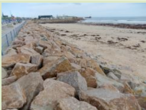
Rock armour in front of walkway with band of yellow lichens. Photo taken looking north north east.
