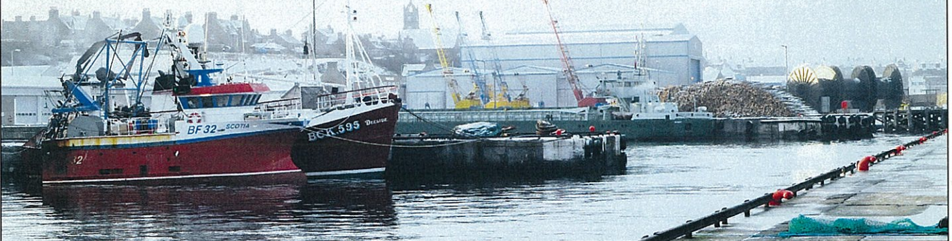
Buckie harbour and the surrounding area could become a bustling hub servicing the Moray Firth offshore renewable energy industry, it was revealed last week.
